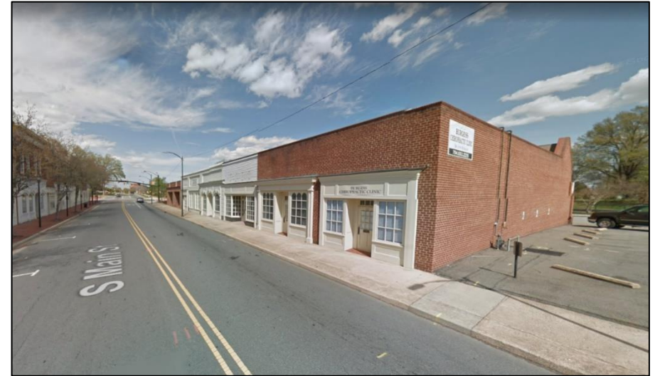
The site from the southwest
